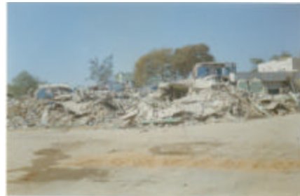
Lanes of Houses destroyed at Bhuj City
